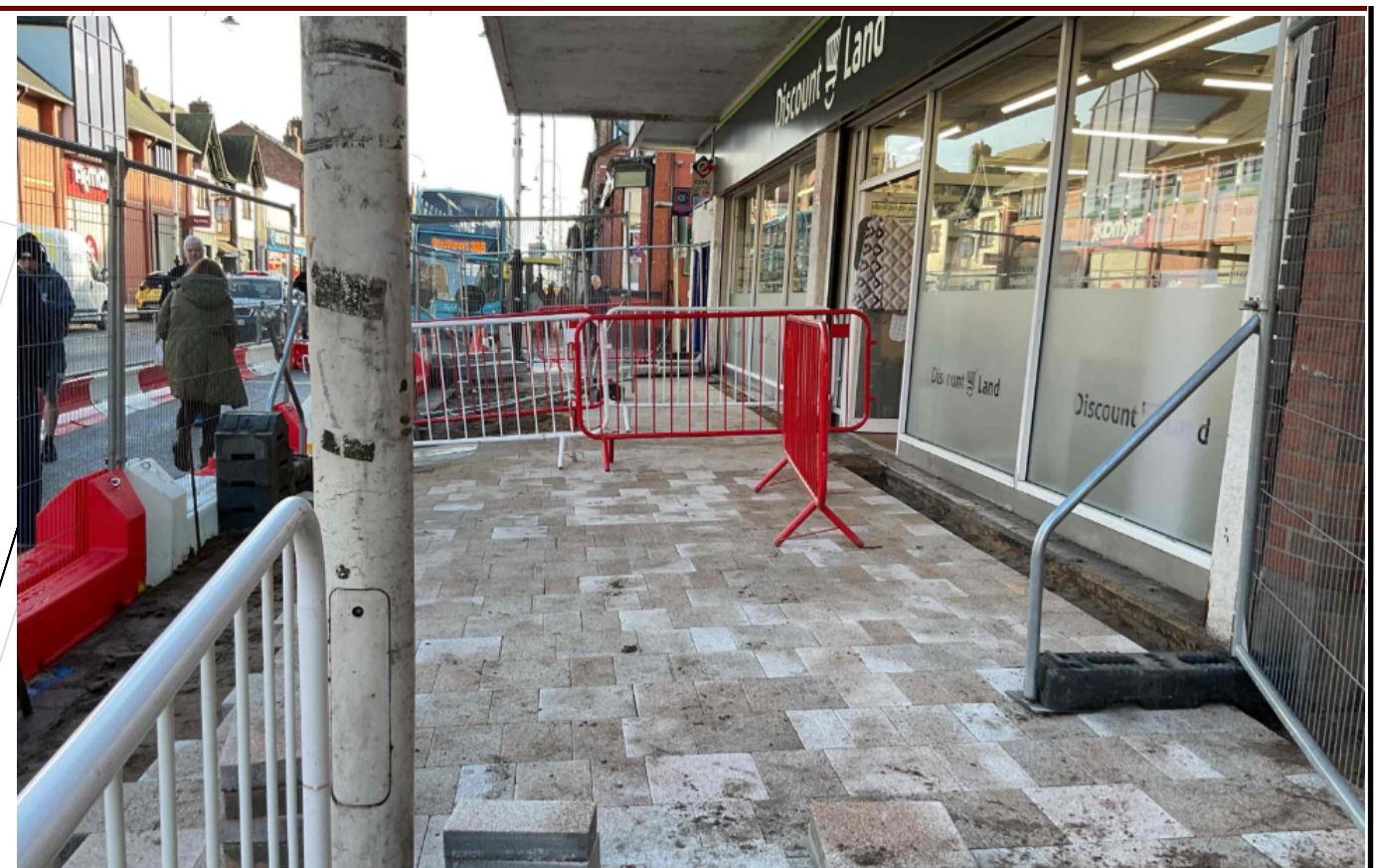
Bus Stop Relocated
